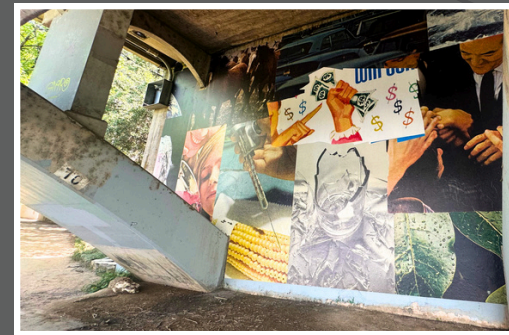
Lamar Blvd Bridge (30.26496, -97.75697)
