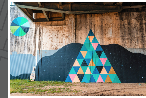
1st Street Bridge (30.26371, -97.74766)
