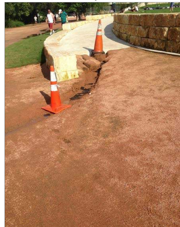
Figure 2.53: Rills can form when proper dispersal mechanism are absent, like this ramp at Auditorium Shores.
